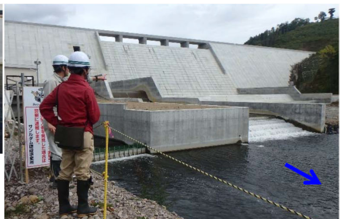
Downstream end of Pool type Fish passage
