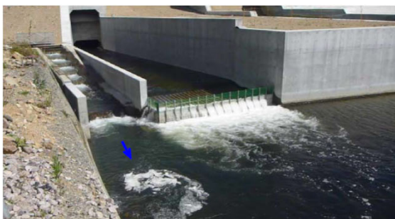
Downstream end of Pool type Fish passage
