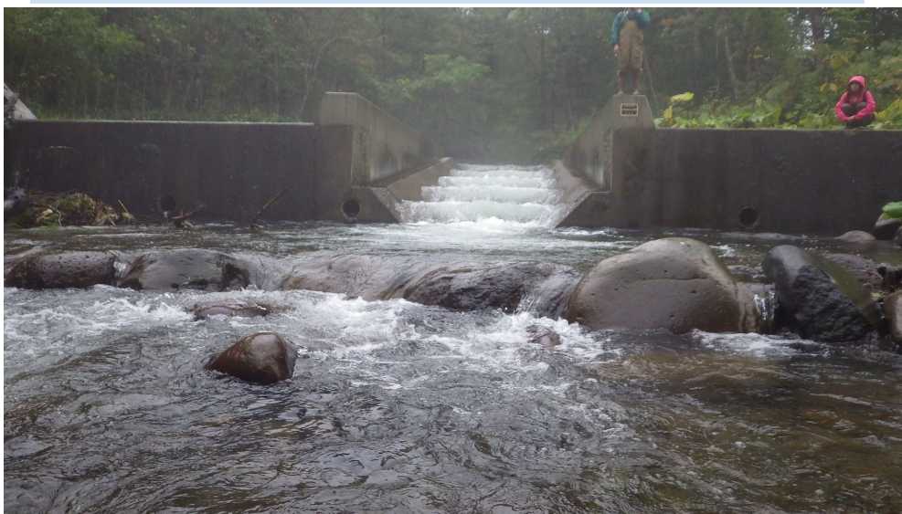
Stacked boulders below check dam with a compound section
