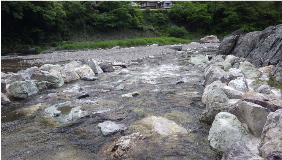
Flow condition in stacked boulders below a fish passage
